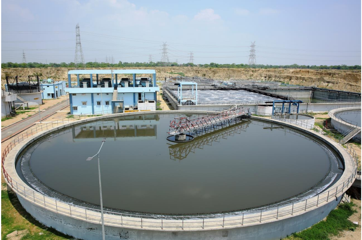
STP PLANT - SOFIPUR VILAGE BLOCK & District Firozabad
